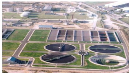
Thessaloniki Wastewater Treatment Plant
